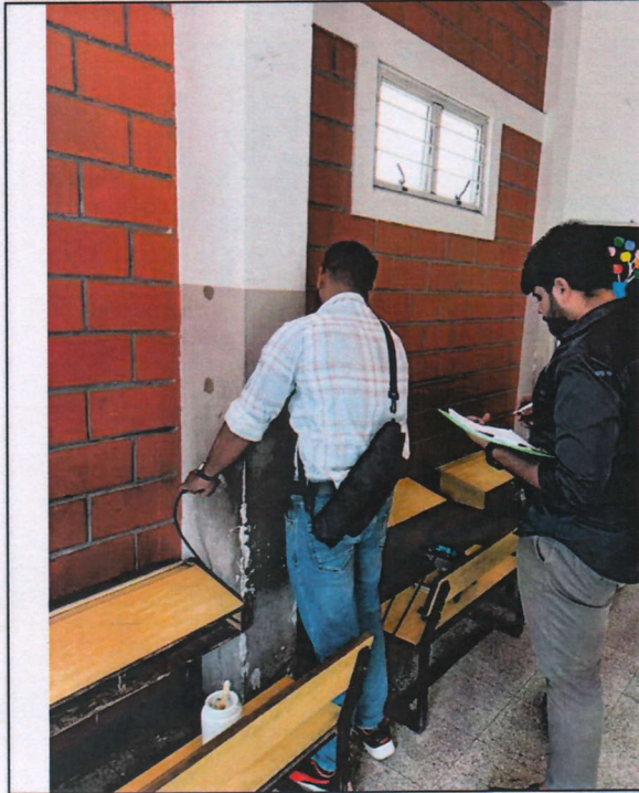
Ultrasonic Pulse velocity test on RC Column
