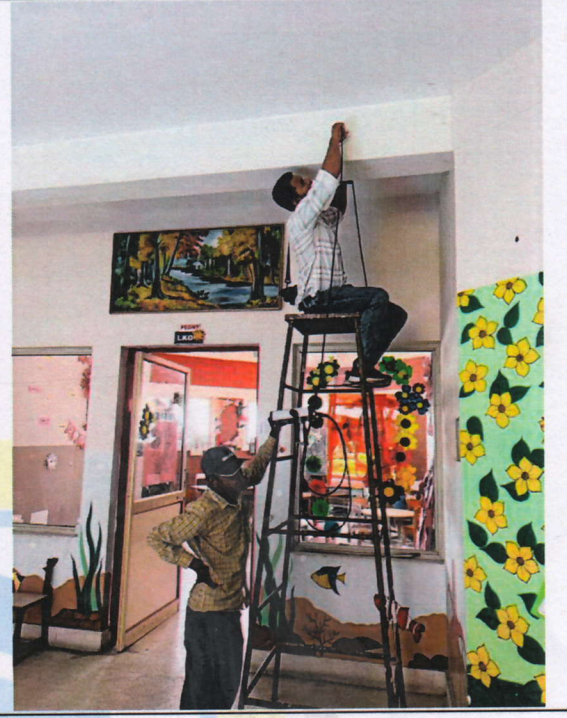
Ultrasonic Pulse velocity test on RC Beam
